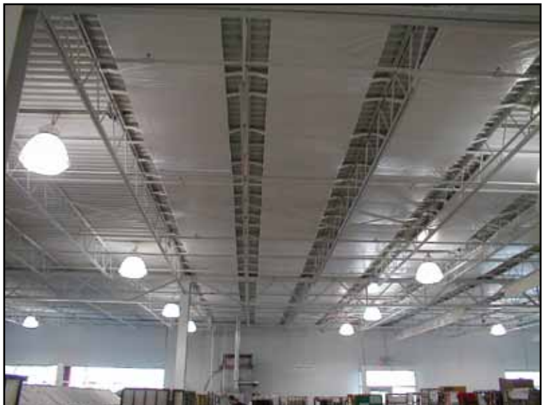
Kinetics model S4 Panel Absorber mounted in the overhead trusses control unwanted reverberant noise to acceptable levels.
