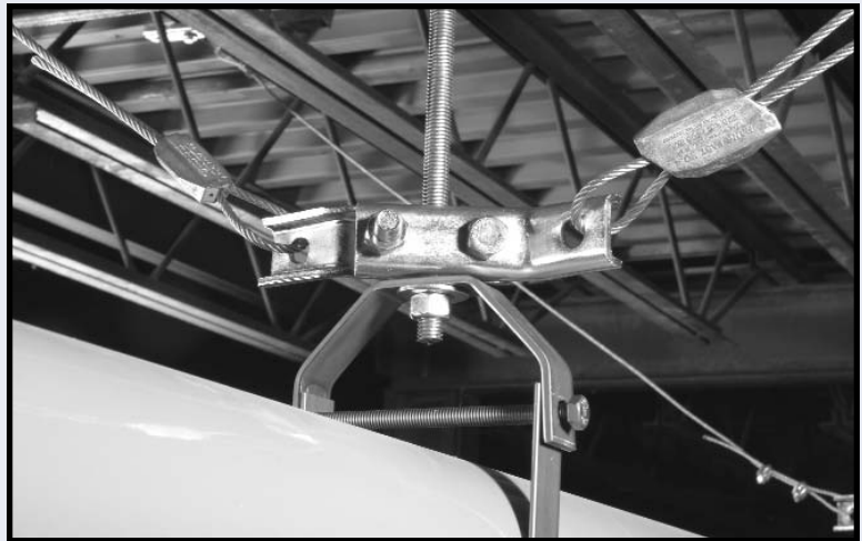
KSCA Hanger Rod Connection with Gripples, (Fig. 2)
