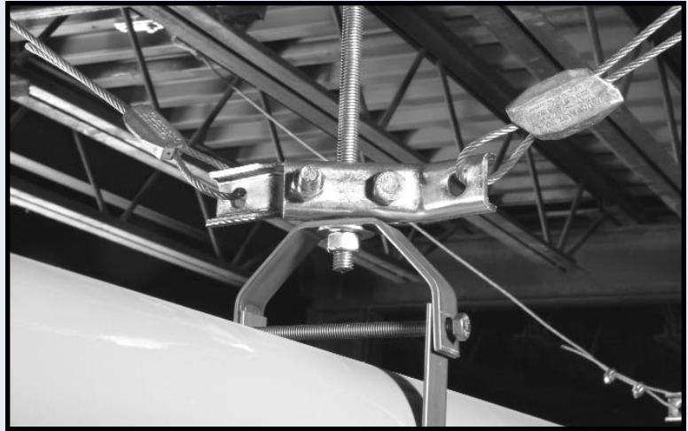
KSCA Hanger Rod Connection with Gripples, (Fig. 2)
